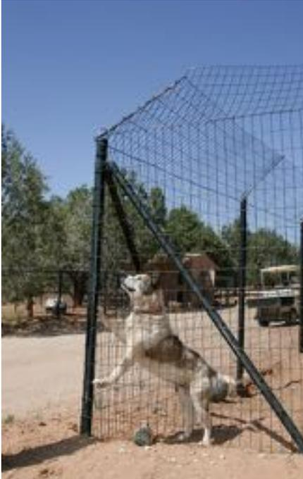
**Top-Angling.** (above) A slightly different approach to the flat-top: Angle the fence extension so that it's aimed upward.
